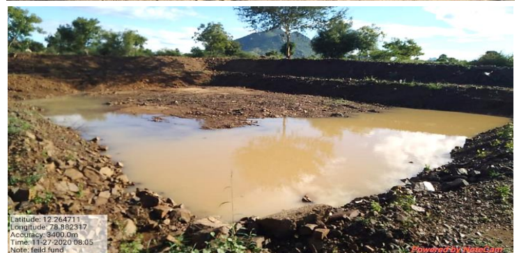
Percolation pond at Melpennathur
